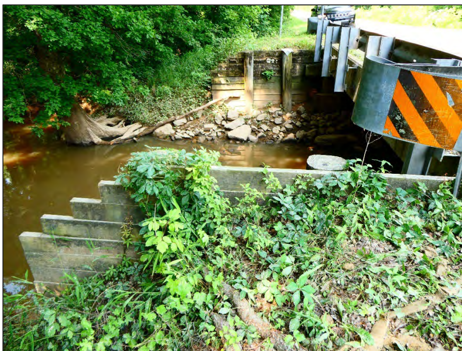
Figure 26: View of Bridge 30, timber pile abutments, facing west from SR-87.
