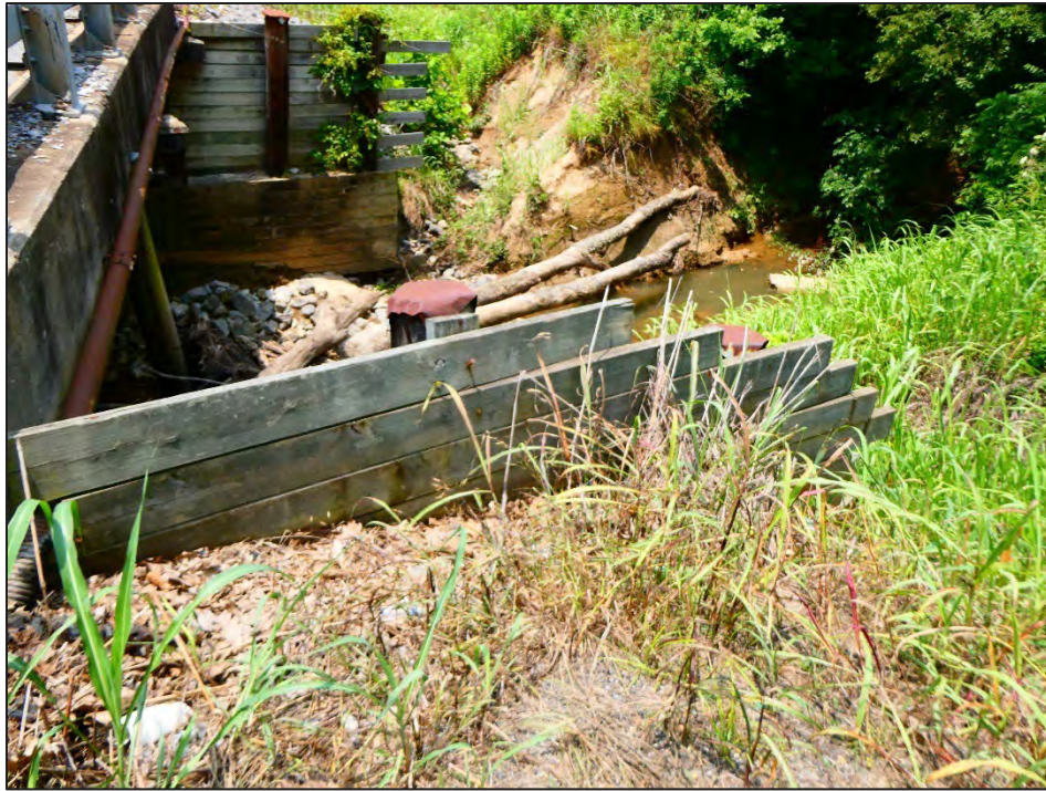
Figure 96: View of Bridge 50, timber pile abutments, facing west from SR-87.
