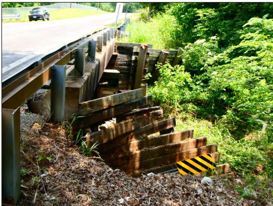
Figure 95: View of Bridge 50, timber pile abutments, facing east from SR-87.
