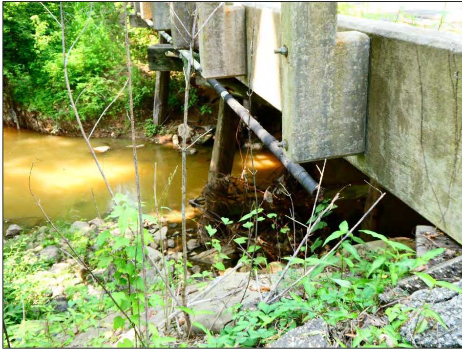
Figure 29: View of Bridge 31, timber pile bents, facing north from SR-180.
