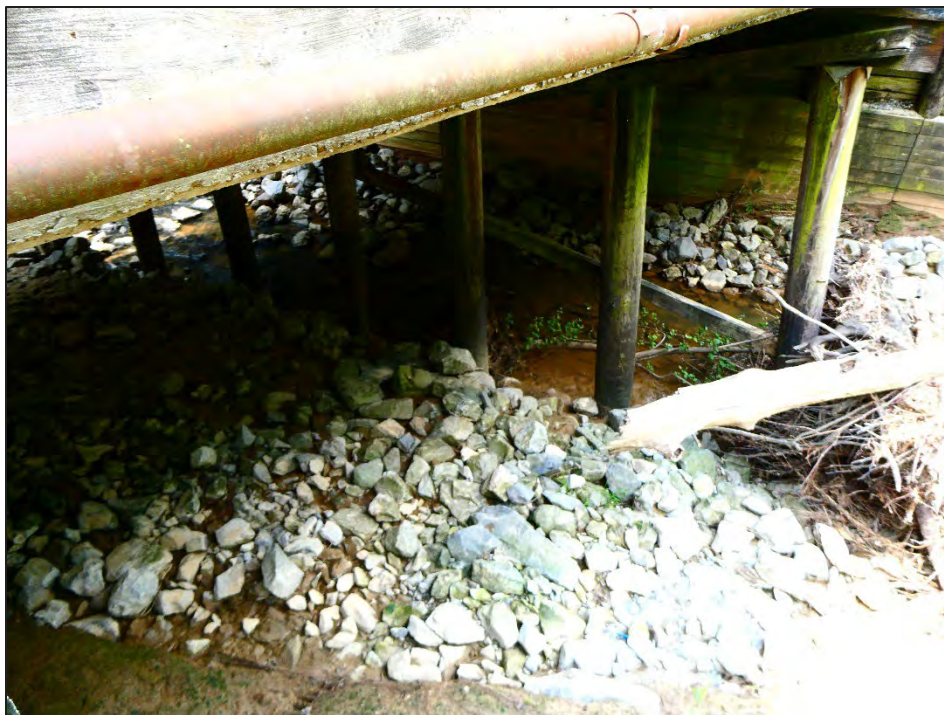
Figure 98: View of Bridge 50, timber pile bents, facing southwest from SR-87.
