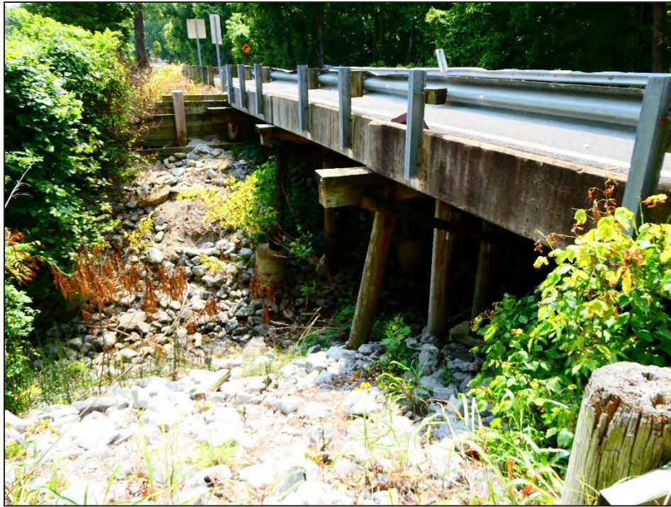
Figure 78: View of Bridge 48, concrete caps, timber pile bents, and timber pile abutments, facing west from SR-87.
