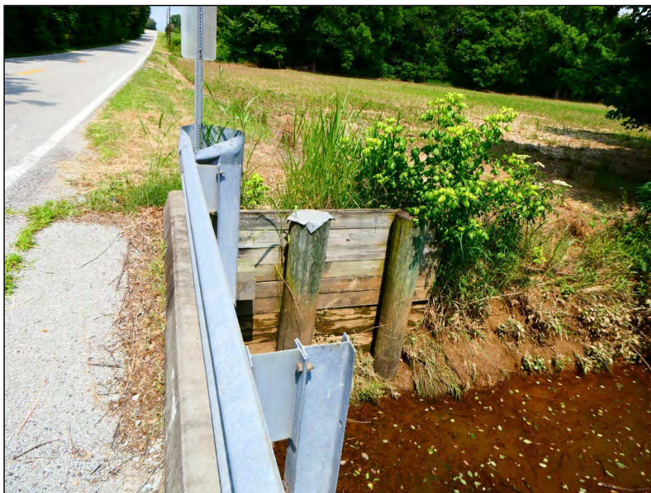
Figure 14: View of Bridge 41, timber pile abutments, facing west from SR-87.
