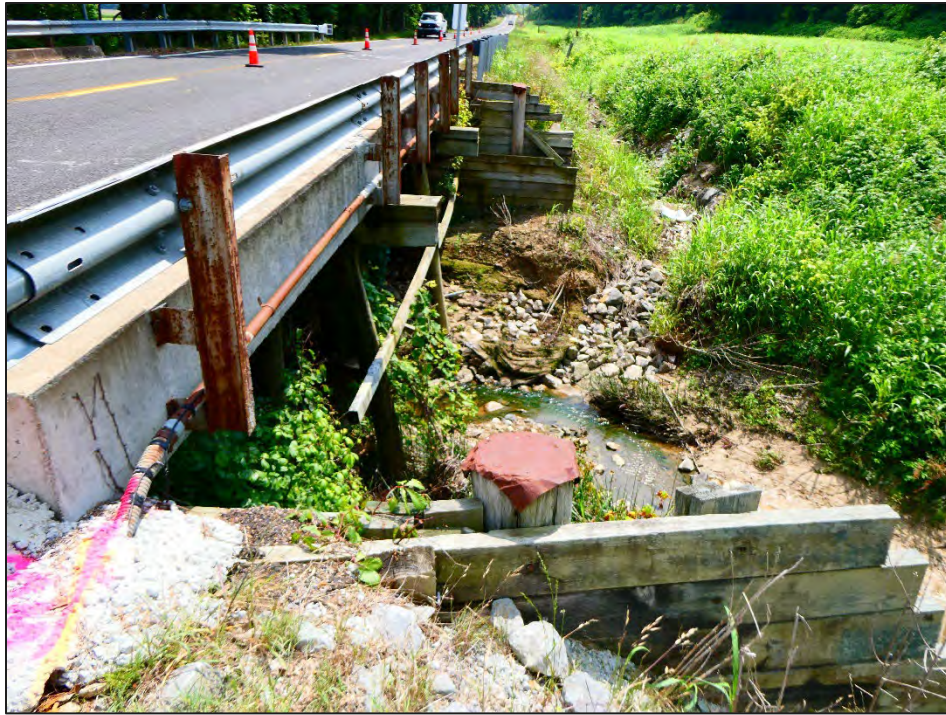
Figure 75: View of Bridge 47, concrete caps and timber pile abutments, facing north from SR-87.
