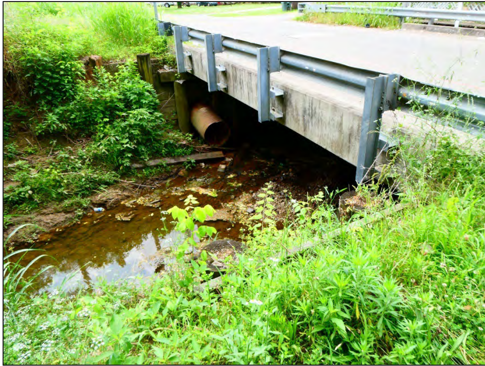
Figure 42: View of Bridge 46, concrete pile caps with metal guardrails and timber pile abutments, facing south from SR-87.
