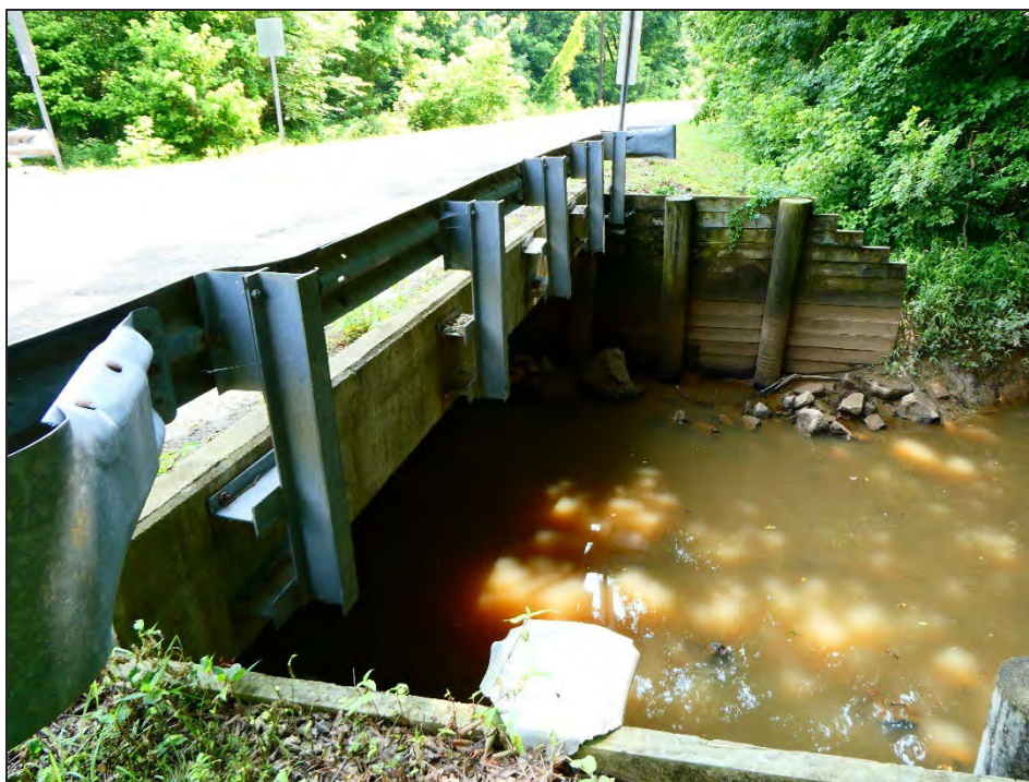
Figure 25: View of Bridge 30, concrete caps and timber pile abutments, facing east from SR-87.
