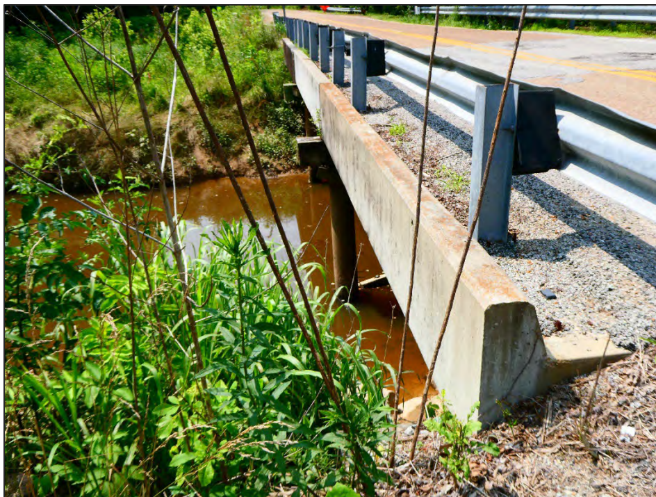
Figure 21: View of Bridge 29, concrete girder and timber bent and piers facing northwest from SR-87.
