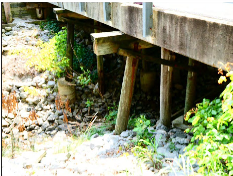
Figure 79: View of Bridge 48, timber pile bents, facing west from SR-87.
