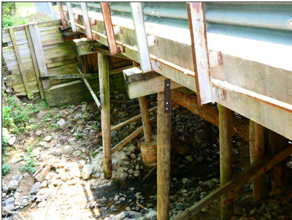
Figure 76: View of Bridge 47, timber bents, facing west from SR-87.
